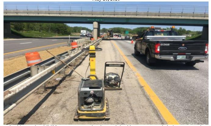
Looking north at MM35, crews are removing damaged shoulder pavement and placing new gravel.
