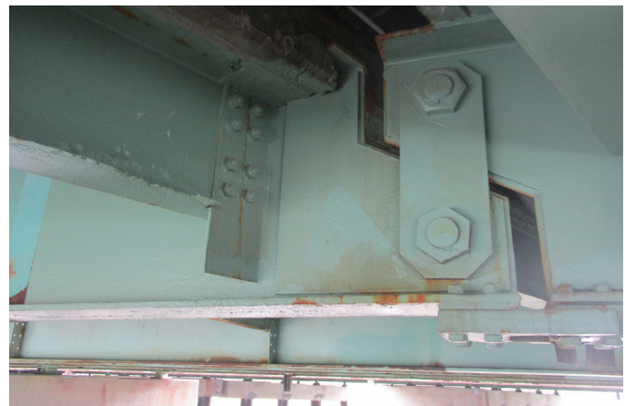
PIN-AND-LINK ASSEMBLY AT THE YORK RIVER BRIDGE
