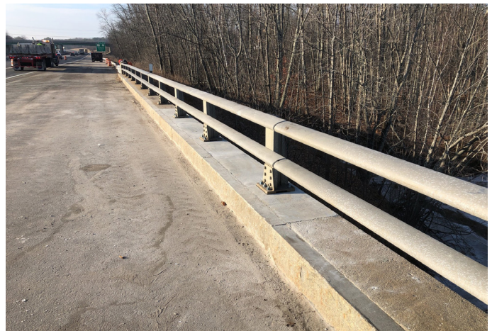
SACO RIVER OVERPASS REPAIRED BRIDGE RAIL
