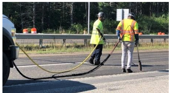
DISPENSED AT OVER 350 DEGREES THE RUBBERIZED ASPHALT SEALANT IS INJECTED DIRECTLY INTO PAVEMENT CRACKS DURING CRACK REPAIRS
