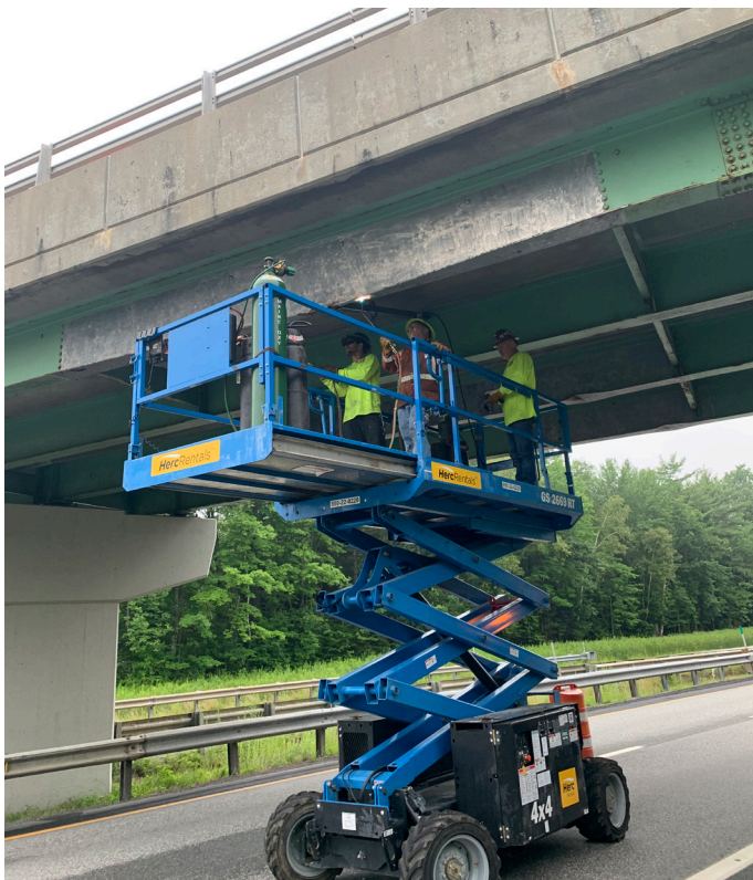
GROVE STREET UNDERPASS, MILE 83.7
