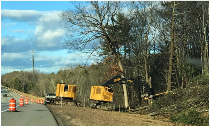
SIDE SLOPE CLEARING
