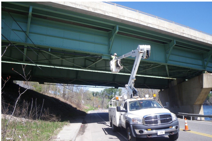
HANDS-ON INSPECTION OF THE ANDROSCOGGIN RIVER BRIDGE
