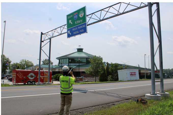
OVERHEAD SIGN STRUCTURE INSPECTION
