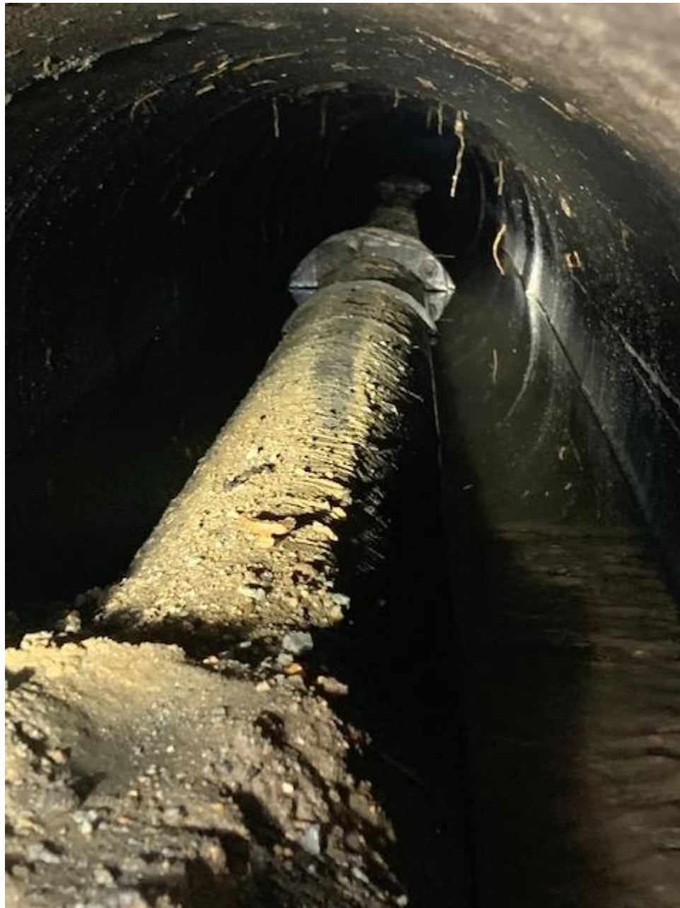
Typical Mechanical Joint (Wood Skids Attached Under Each Joint)
