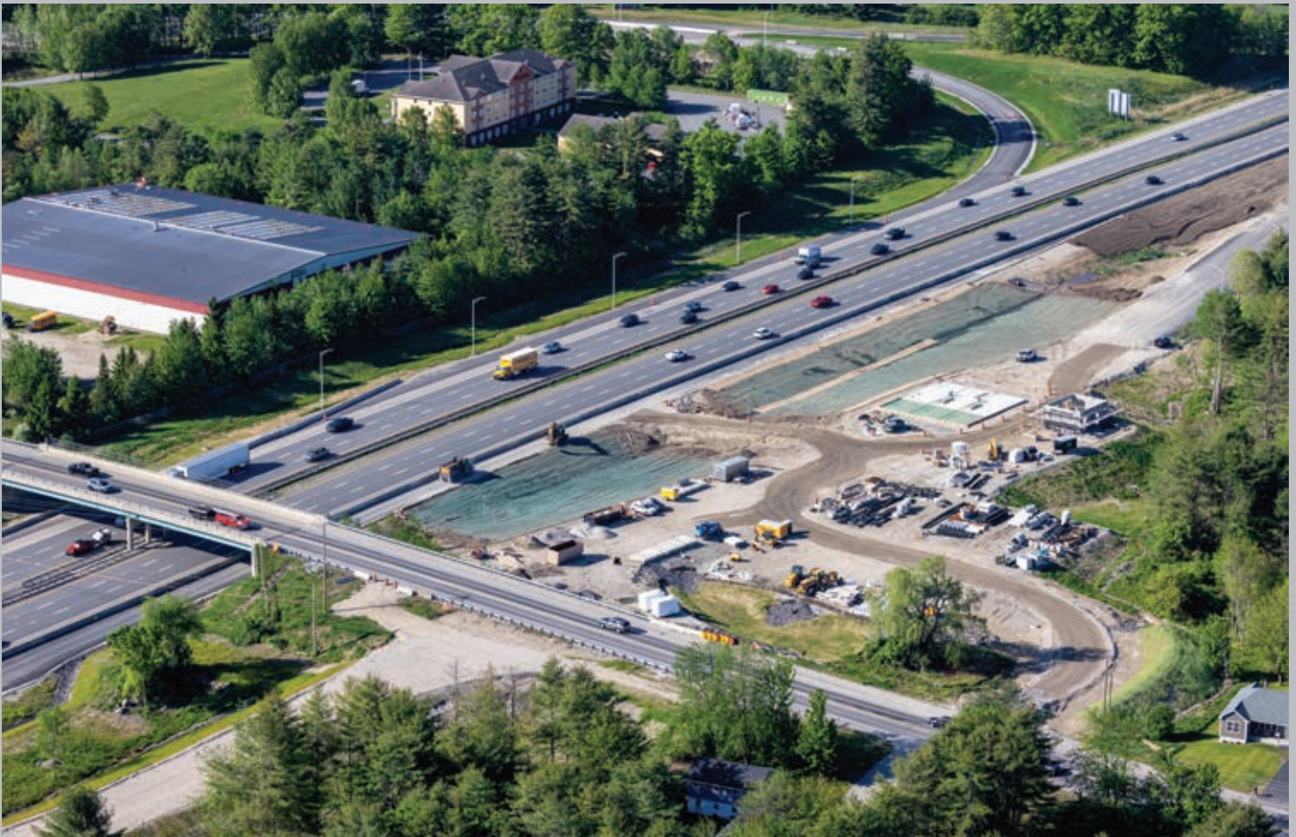
The new southbound on-ramp and toll plaza area at Exit 35 in Saco in May 2024.
