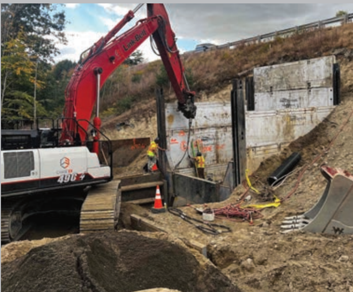
Crews use equipment to rebuild the slope in Auburn in October 2024
