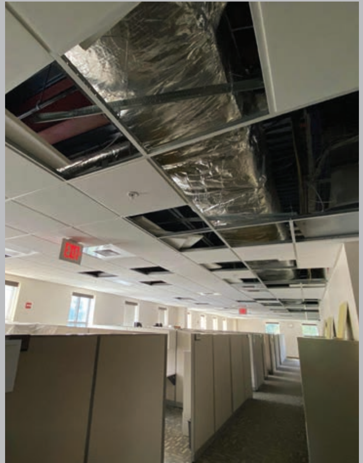
Ceiling tiles at MTA headquarters awaiting new LED lighting in August 2024
