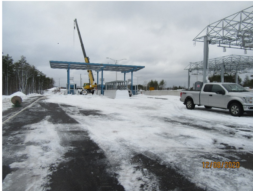
Erecting NB cash lane canopy
