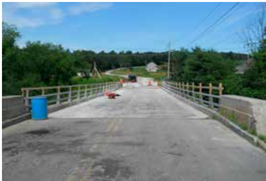
HURRICANE ROAD OVER PISCATAQUA RIVER
