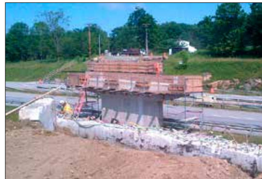
OLD LISBON ROAD UNDERPASS
