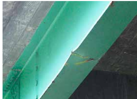
GODDARD ROAD SOUTHBOUND OVERPASS, MILE 79.6
