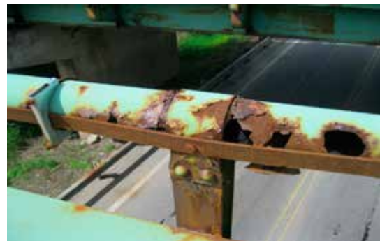
LEWISTON INTERCHANGE "PORK CHOP" BRIDGE RAIL
