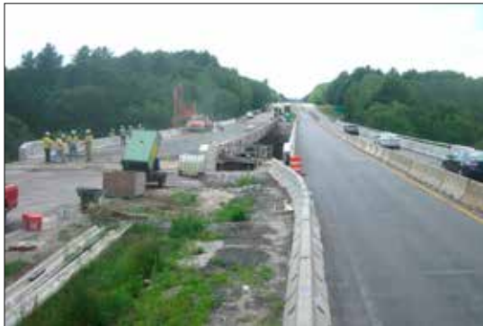
PRESUMPCOT RIVER BRIDGE OVERPASS
