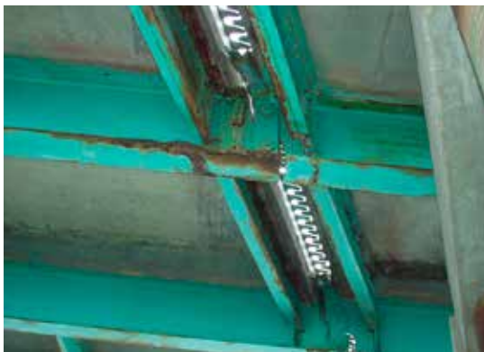
PIN-AND-HANGER ASSEMBLY AT THE YORK RIVER BRIDGE
