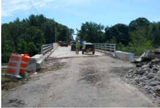
HURRICANE ROAD UNDERPASS
