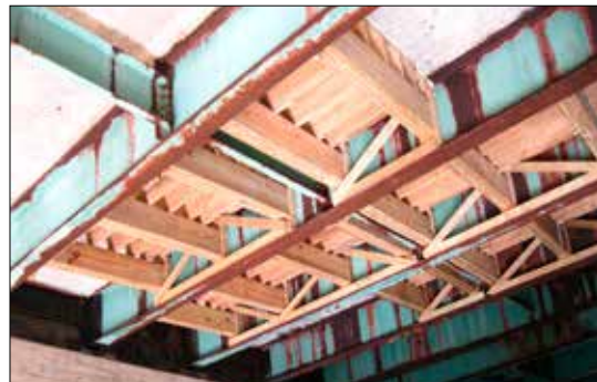
PISCATAQUA RIVER STRUCTURE #31
