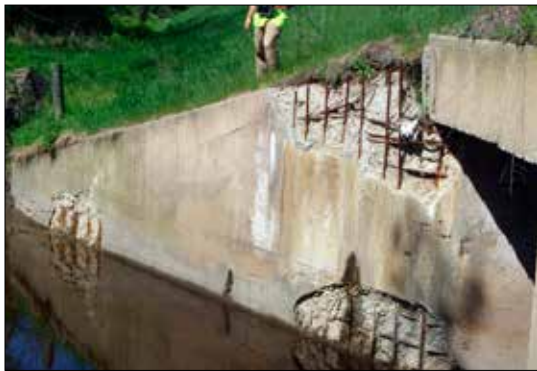
NO-NAME RIVER CULVERT
