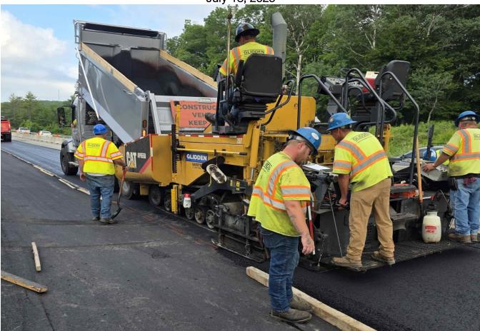
Crews work on finishing the median cross overs that will be used by the end of summer to allow for bridge joint replacements.
