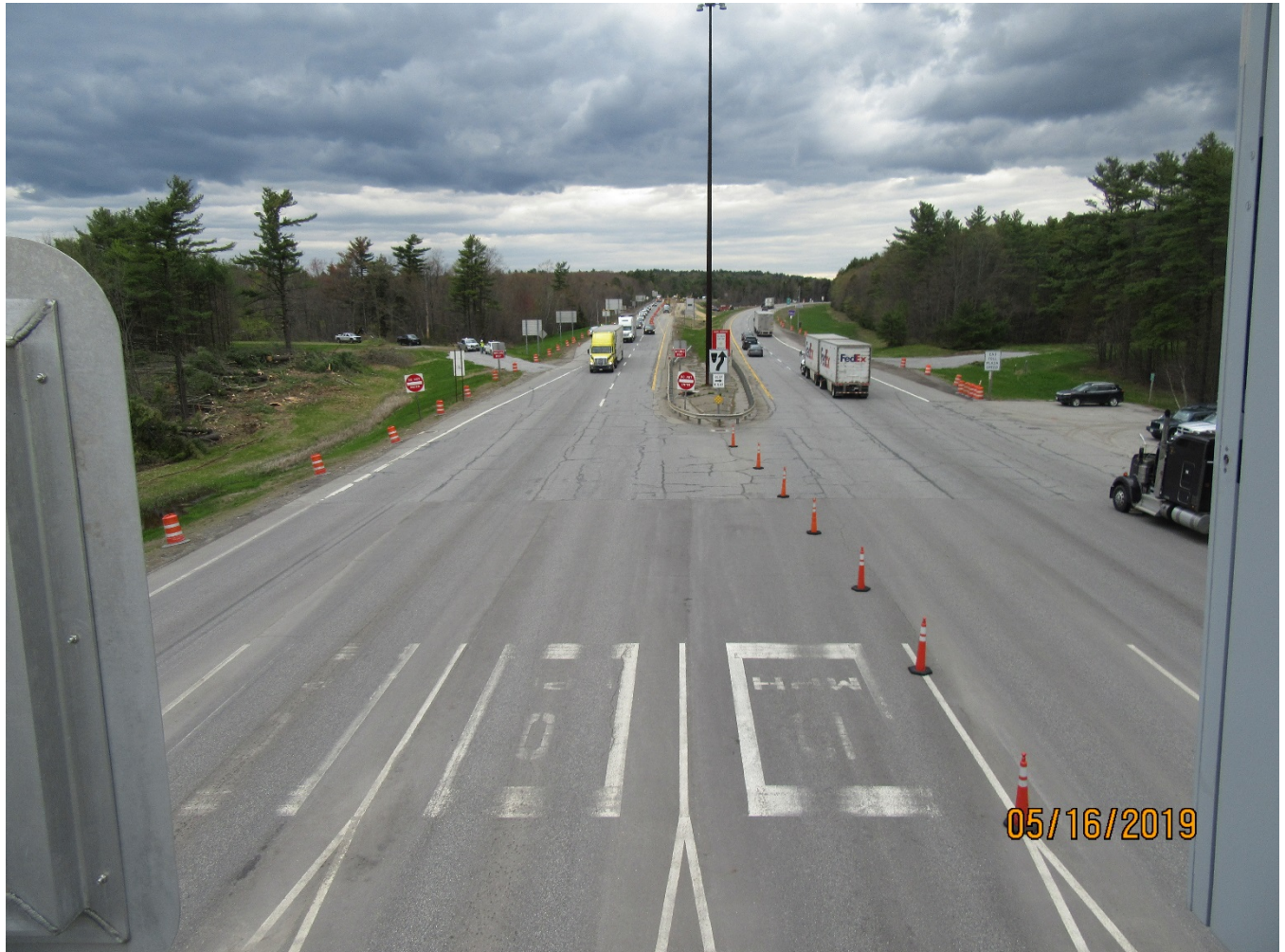
Future location toll plaza just north of the existing
