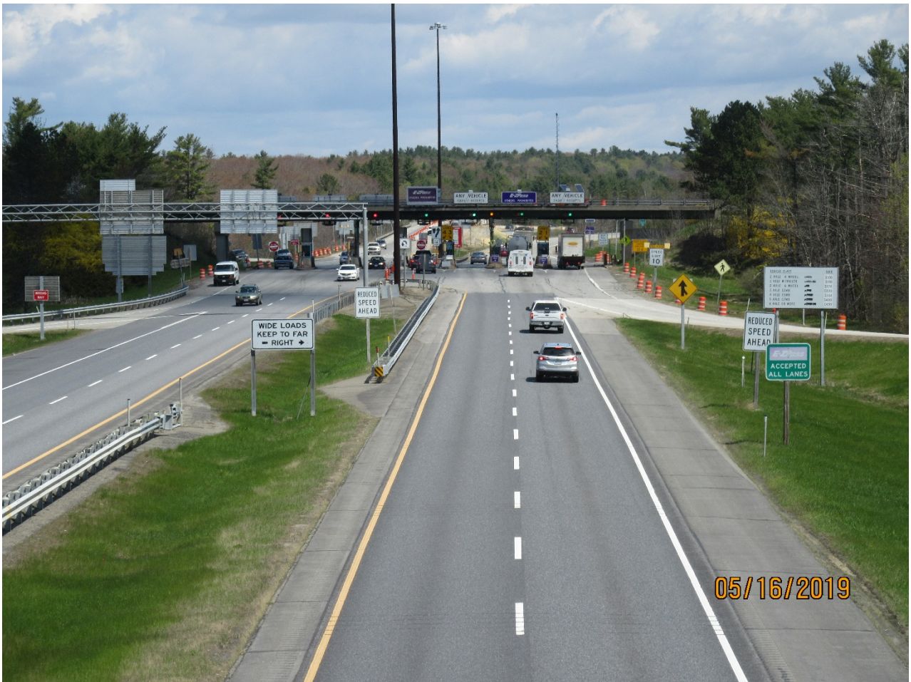
Existing west Gardiner plaza
