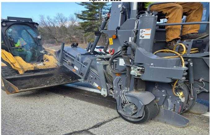
The contractor removes the rumble strips so the shoulder can be made smooth and used for traffic while the bridge is being repaired.
