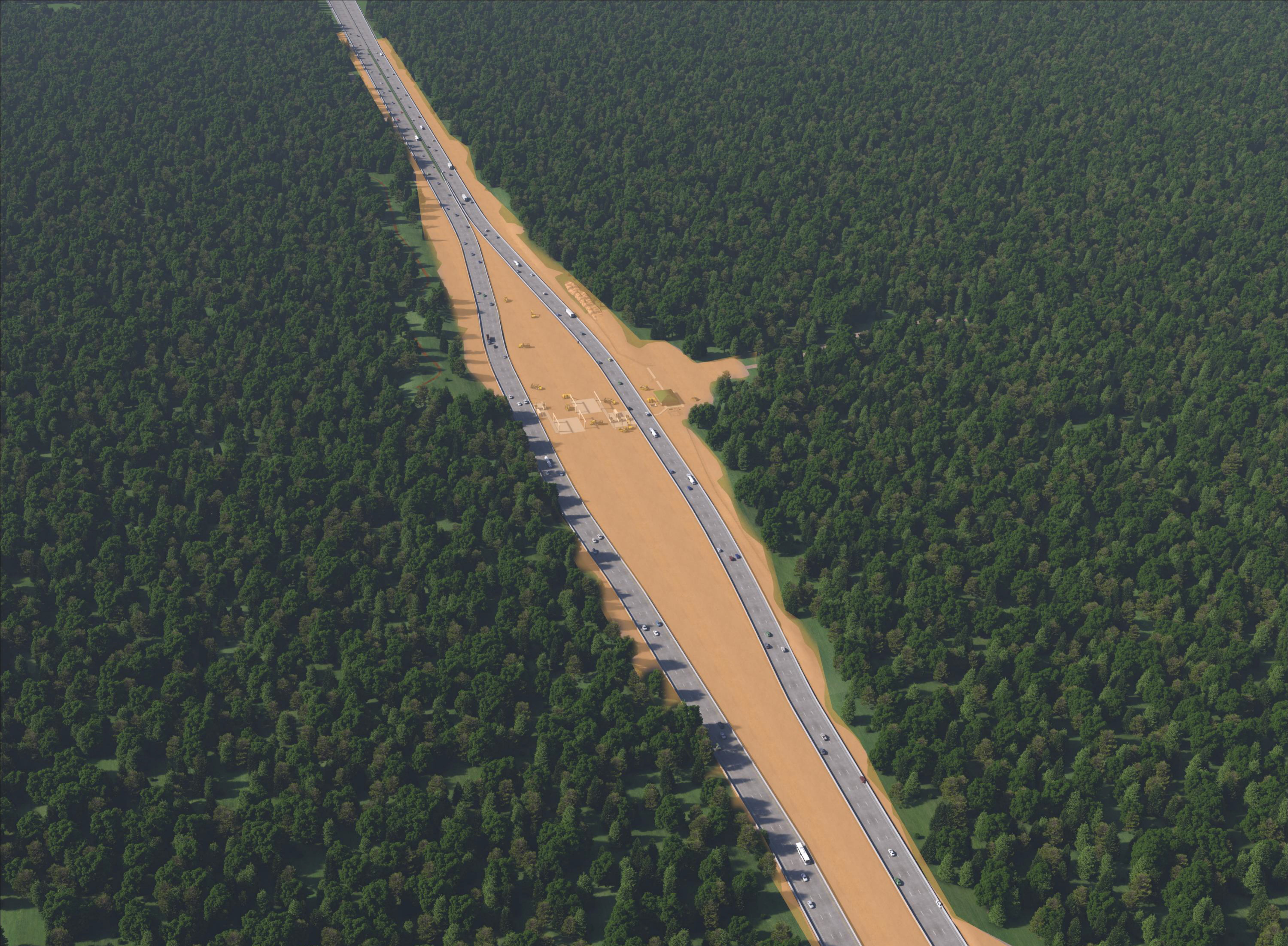
York Toll Plaza at Mile 8.8 - Stage 2
