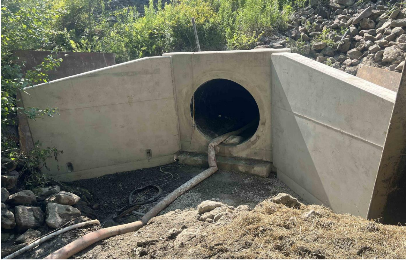
Outlet of the crossing at Mile 40.30 with the new headwall
