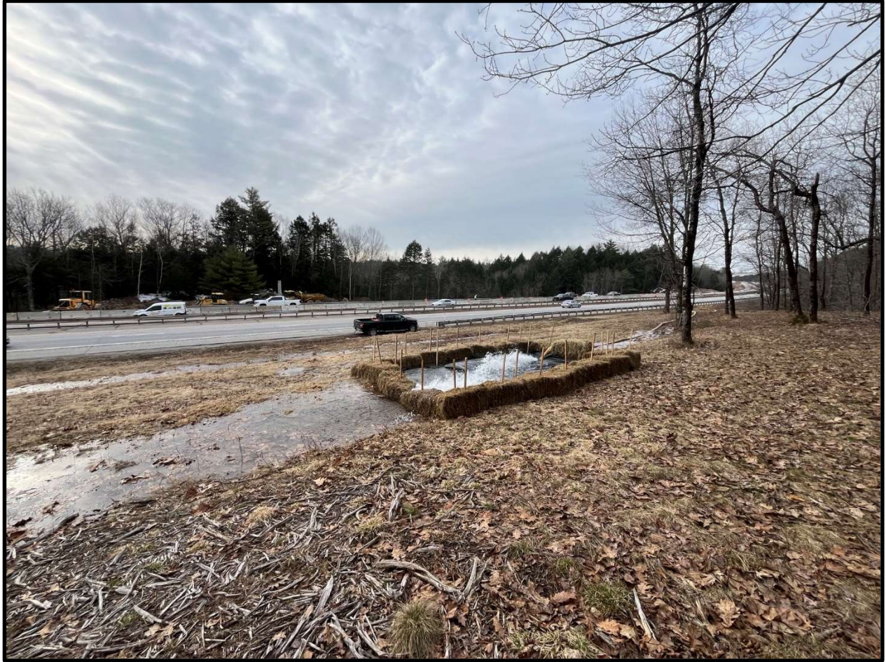
Figure 5 – Southbound hay-bale and filter fabric settlement area. Outfall drains to north away from inlet
