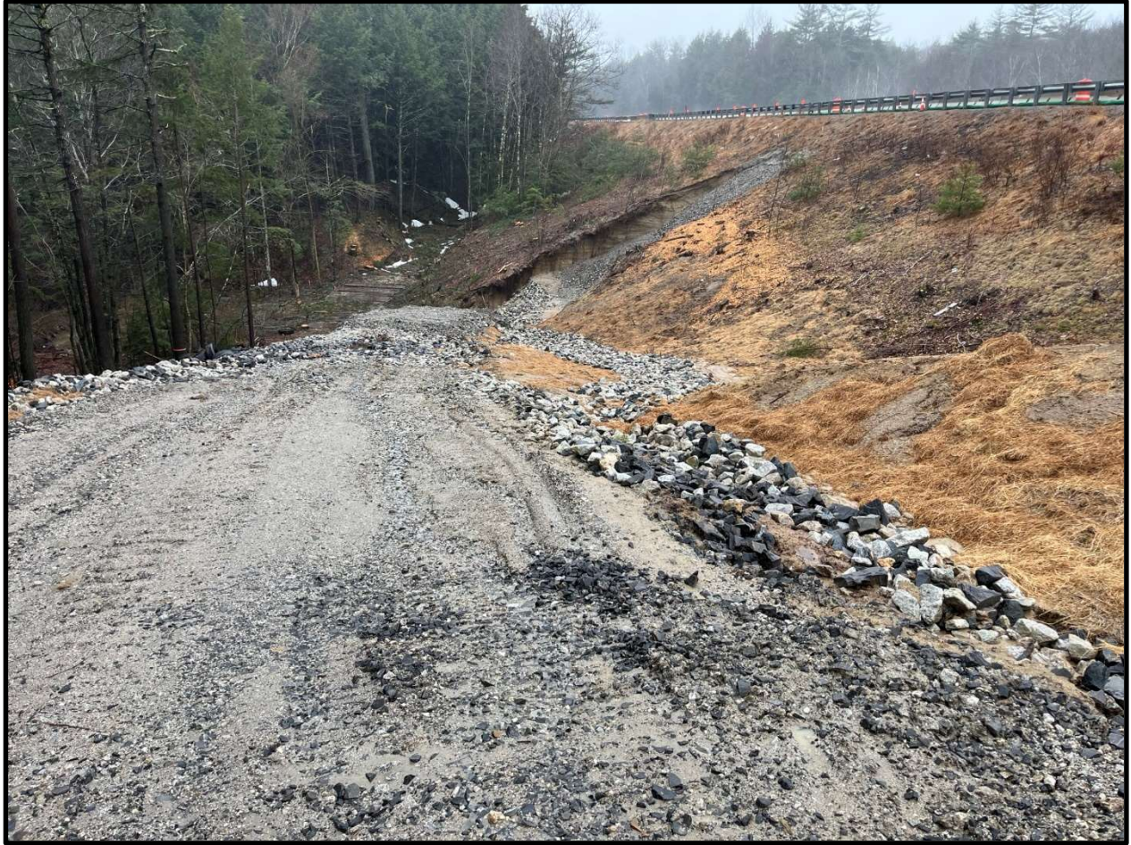
Figure 3 - Northbound Access Road, facing South. Access road to remain.
