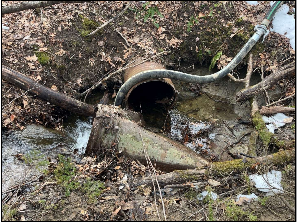
Figure 4 – Southbound Culvert inlet, existing condition (bypass pump from stabilization effort shown.)
