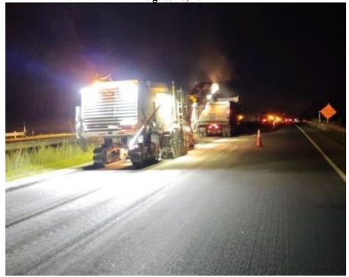
Looking north along the northbound passing lane, crews are crack sealing prior to final paving.
