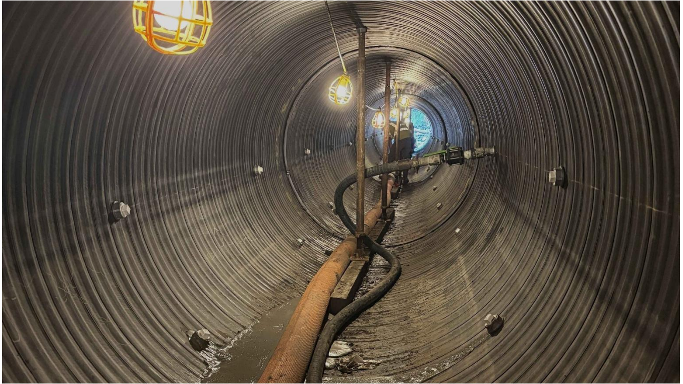
Contractor grouts the annular space between liner and host culverts at Mile 45.9.
