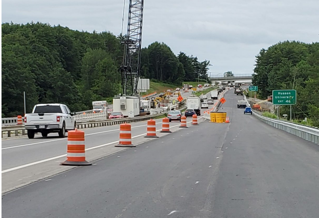
Stroudwater southbound phase 1 paved
