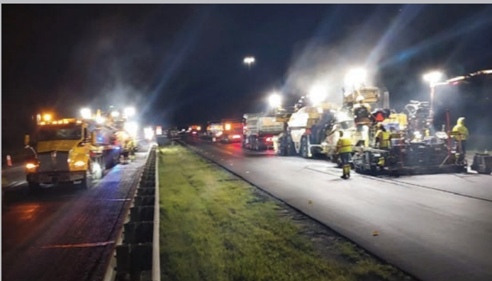
Two crews paving the northbound and southbound lanes in Kittery in October 2024
