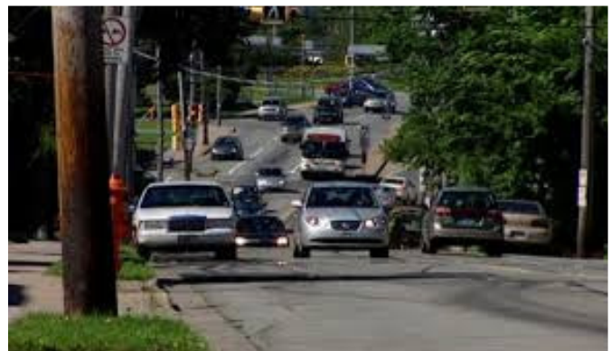
Typical 4-lane roadway – ‘Anywhere U.S.A; Source: Internet
