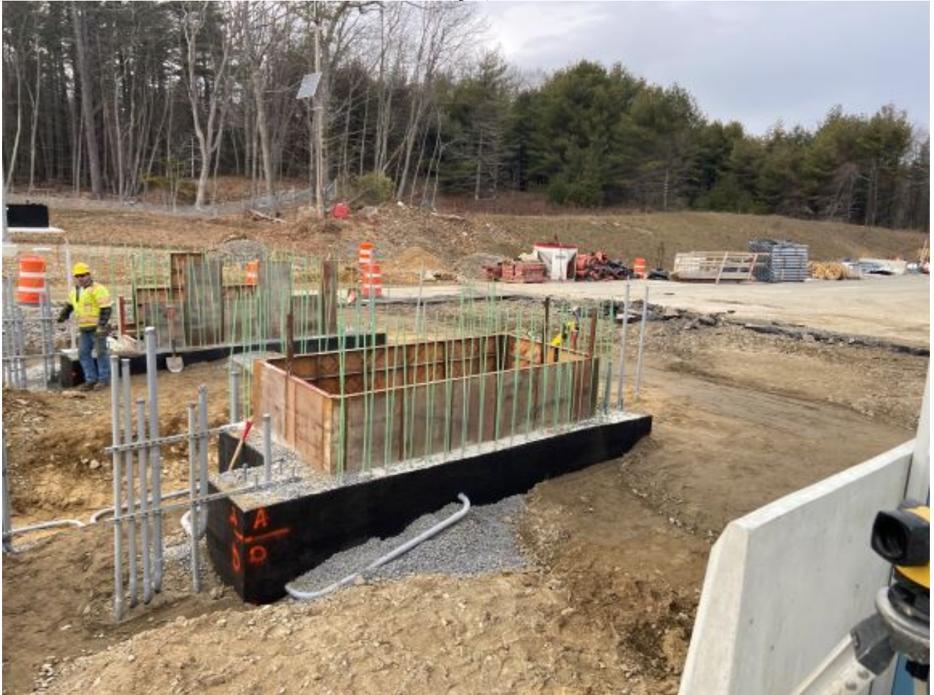
Crews working on forming booths for lanes 1 and 2, southbound.
