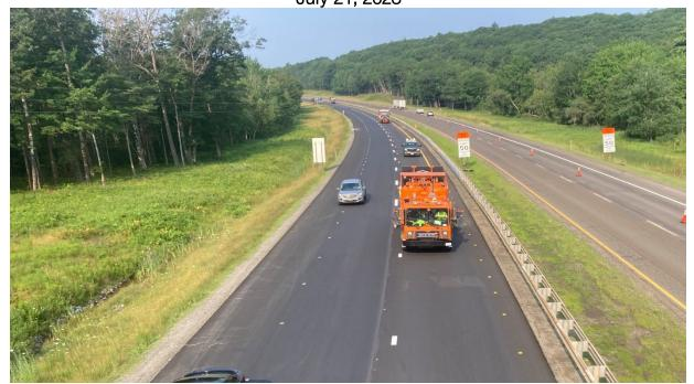
Looking south at the northbound lane, an MTA line striper applies permanent striping to the newly resurfaced roadway.
