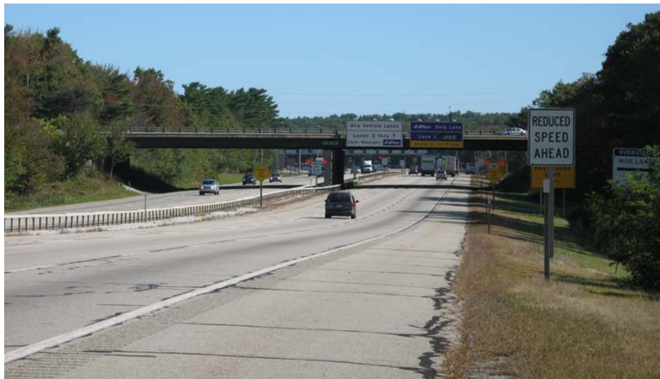
Figure 1 Northbound Sight Distance Bridge and Horizontal Curve Negatively Impact Sight Distance
