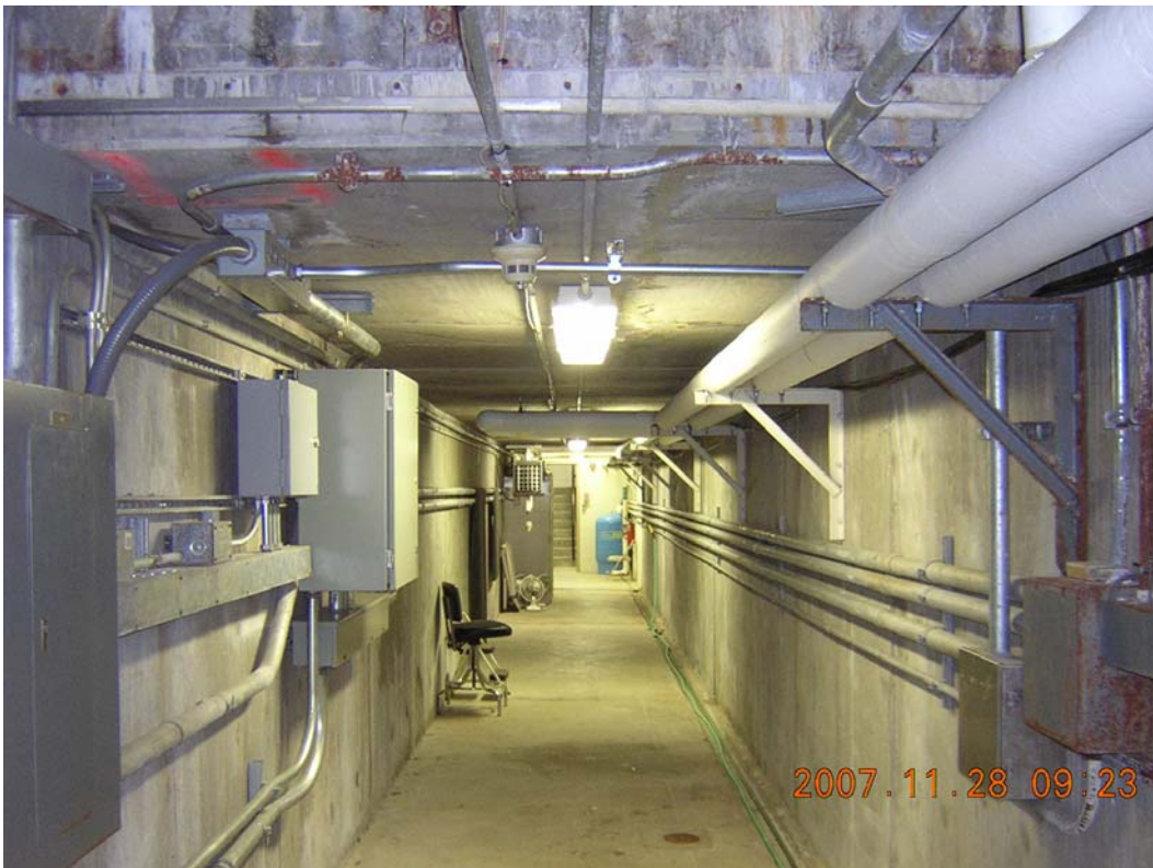
Figure 7 New Gloucester Tunnel
