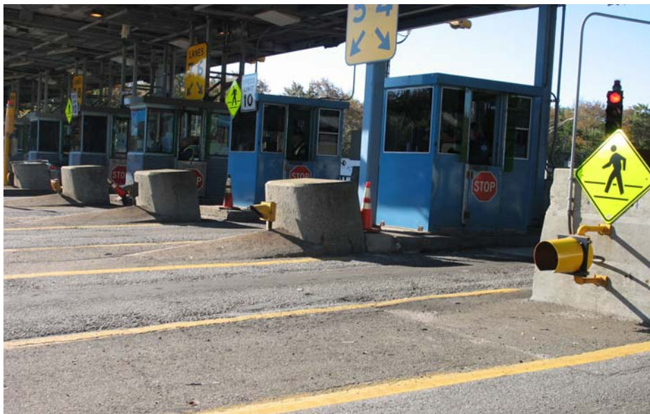
Figure 4 York Toll Booth, Single Bumper and Settled Island
