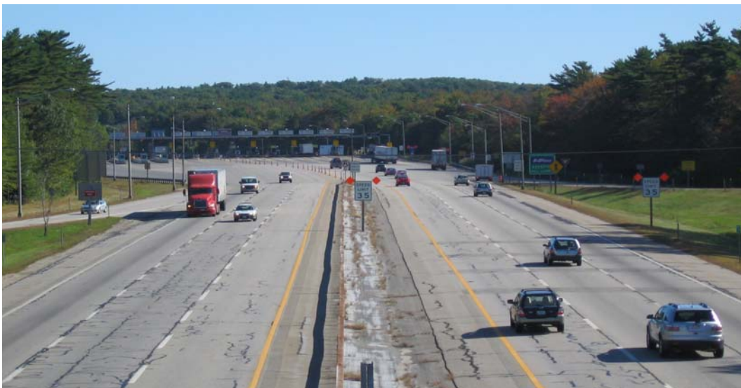
Figure 3 Exit 7 Interchange Ramps South of York Toll Plaza
