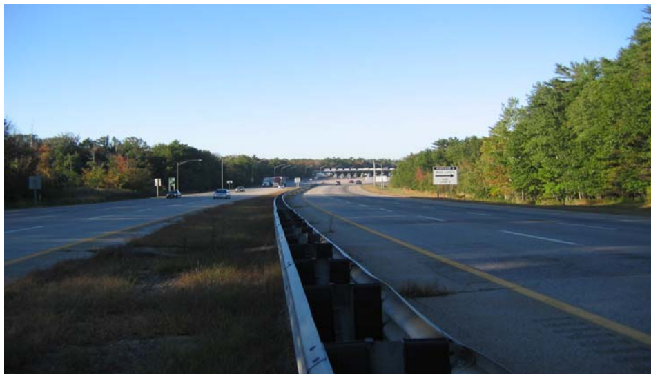
Figure 2 Southbound Sight Distance Horizontal Curve and Down Gradient Are Not Desirable Due To Safety and Operational Concerns
