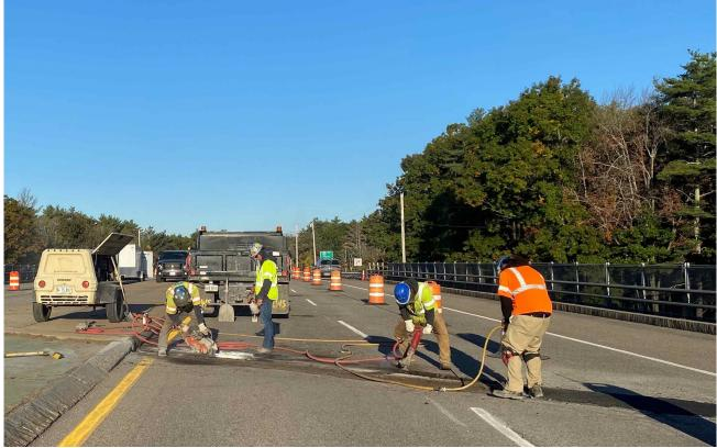
Crews are removing the old joint prior to installing the new one.
