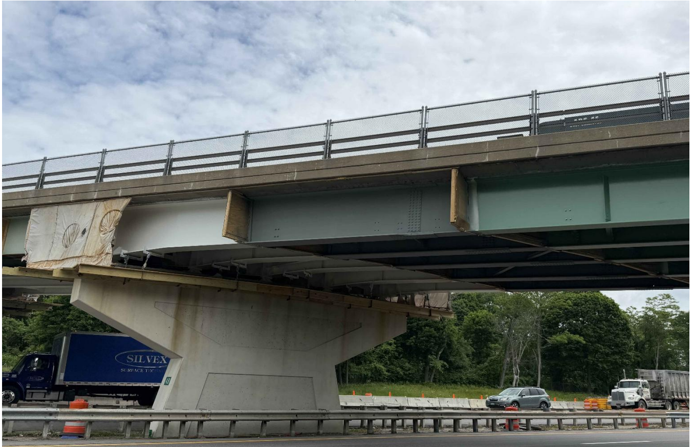
Beech Ridge Road, looking north at the 3-coat system.
