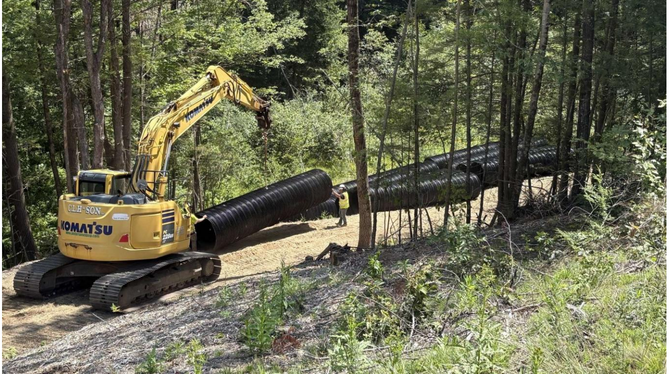
Culvert Slip liner material delivery to Mile 72.0 culvert (Northbound).
