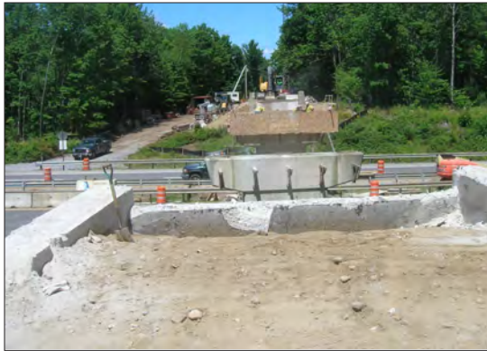
WEST ROAD UNDERPASS, MILE 91.0
