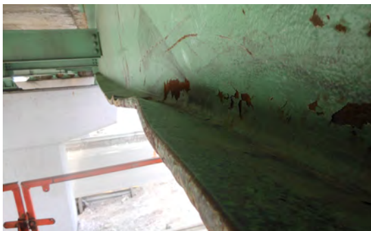
DUTTON HILL ROAD UNDERPASS, MILE 59.9
