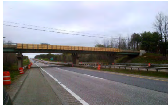
LITCHFIELD ROAD UNDERPASS, MILE 106.9
