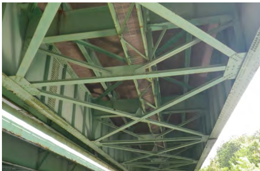
ANDROSCOGGIN RIVER BRIDGE
