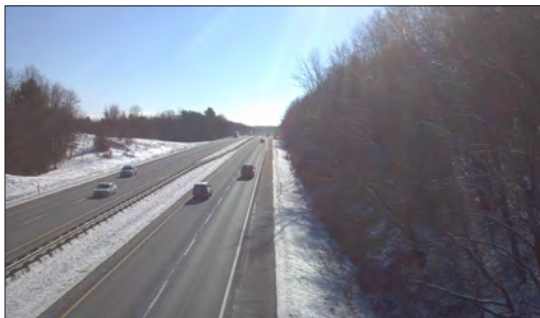
Mile 53.4, Looking South (Before)
