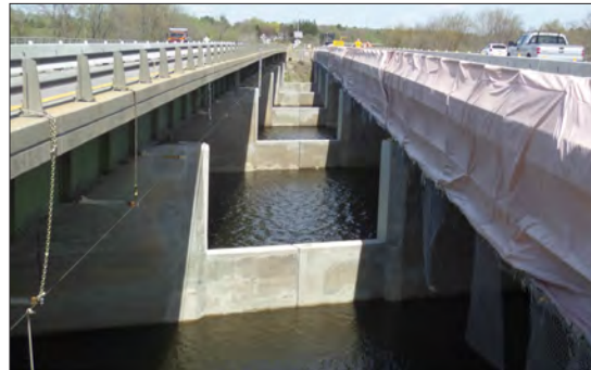
SACO RIVER OVERPASS BRIDGE PAINTING, MILE 33.0
