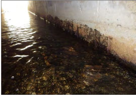
CAPE NEDDICK RIVER BOX CULVERT, MILE 9.6
