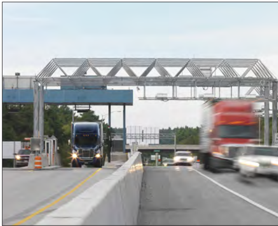
NEW GLOUCESTER TOLL PLAZA
