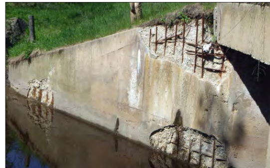
NO-NAME RIVER BOX CULVERT, MILE 82.5
