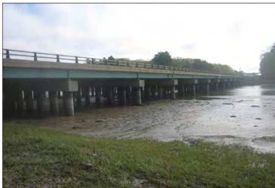
YORK RIVER OVERPASS, MILE 5.2
