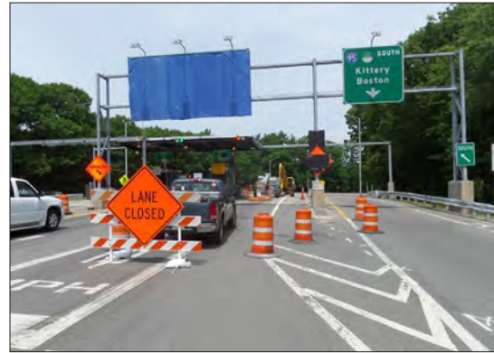
EXIT 19 TOLL PLAZA
