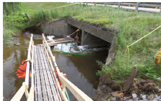
VAUGHAN BROOK BOX CULVERT, MILE 106.94
