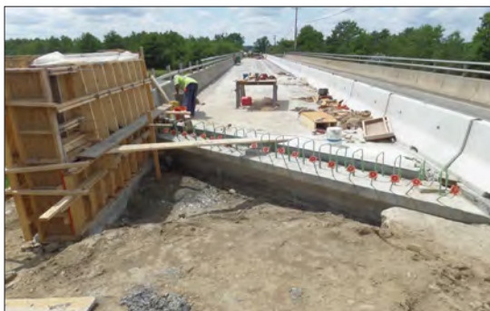
ROUTE 126 UNDERPASS, MILE 101.7
