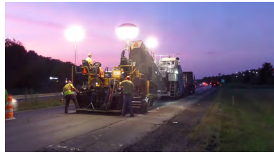
PAVEMENT REHABILITATION MM 102.6 TO MM 109.1
