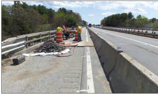
STROUDWATER RIVER OVERPASS, MILE 46.7
