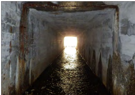
JOSIAS RIVER BOX CULVERT, MILE 11.8
