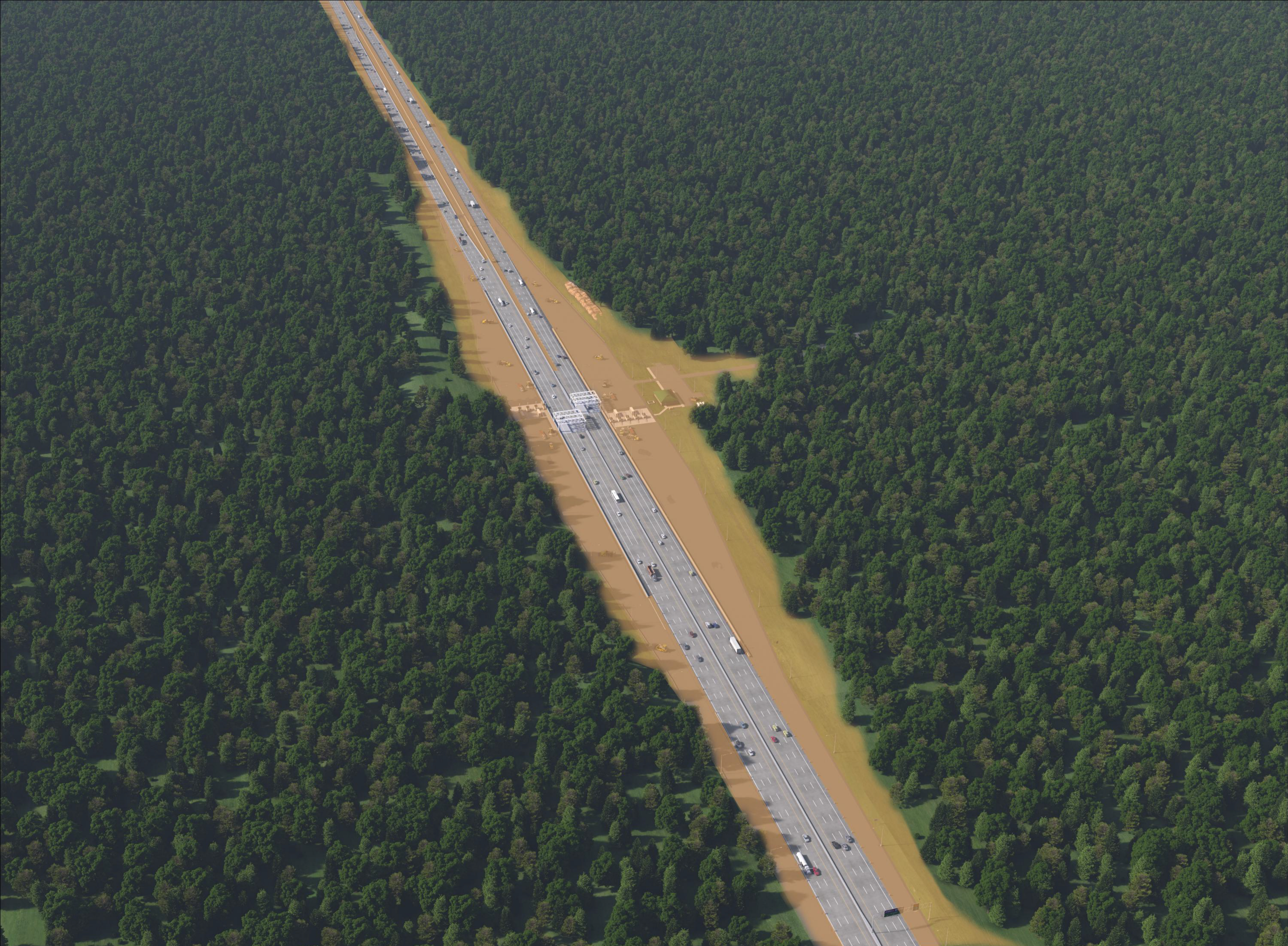
York Toll Plaza at Mile 8.8 - Phase 3
