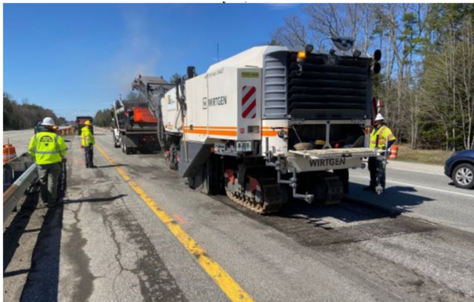
MILLING OPERATION TO PREPARE EXISTING PAVEMENT TO RECEIVE NEW PAVEMENT
