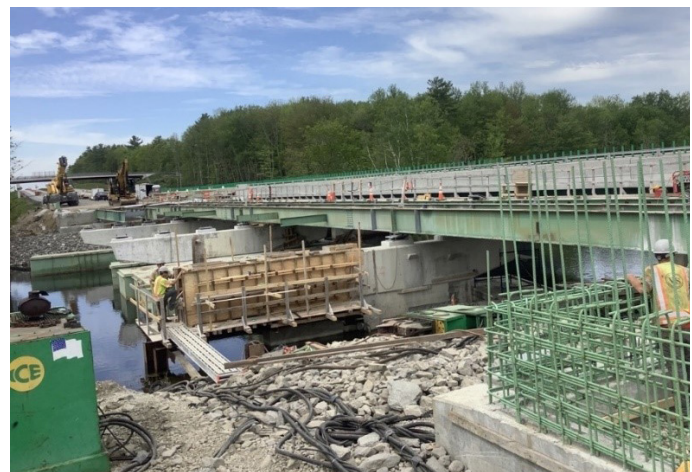
COBBOSSECONTEE STREAM OVERPASS (NB) MILE 99.2
