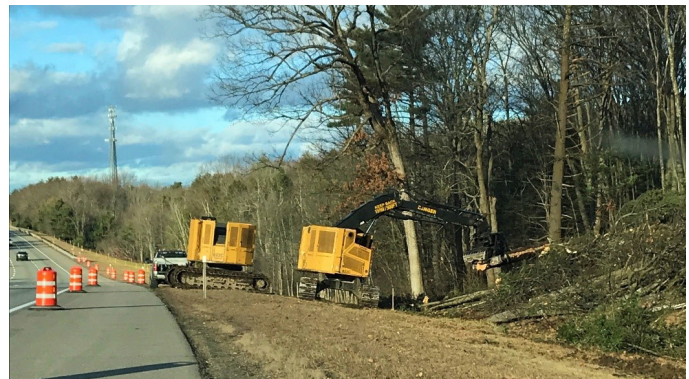
SIDE SLOPE CLEARING
