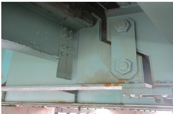
PIN-AND-LINK ASSEMBLY AT THE YORK RIVER BRIDGE
