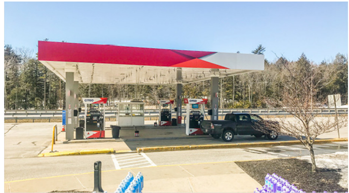
KENNEBUNK SERVICE PLAZA FUEL SYSTEM
