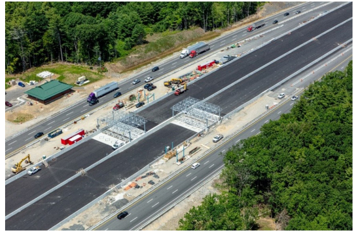
REPLACEMENT YORK TOLL PLAZA
