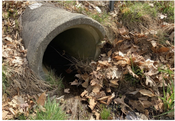
ROADWAY DRAINAGE CULVERT
