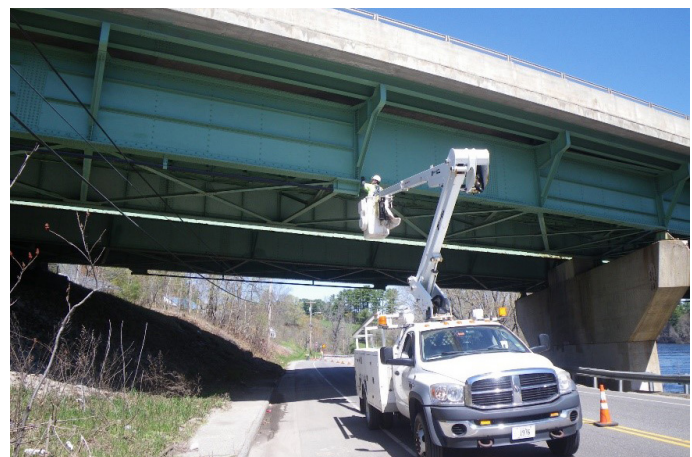
HANDS-ON INSPECTION OF THE ANDROSCOGGIN RIVER BRIDGE
