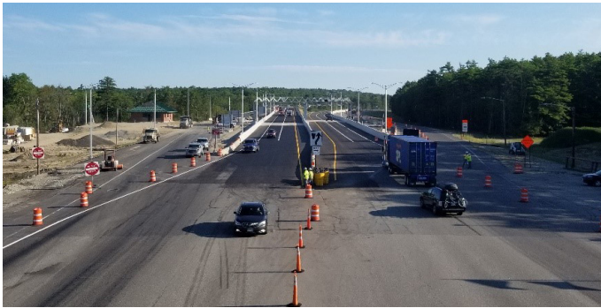
WEST GARDINER I-295 TOLL PLAZA REPLACEMENT
