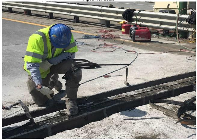
The contractor is removing portions of the old bridge joint in preparation for repairs
