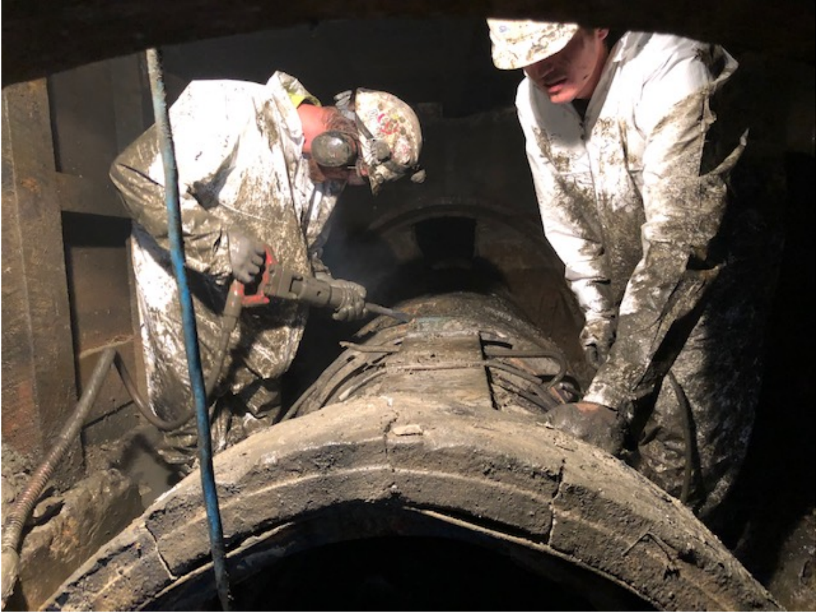
Repairing existing water line casing
