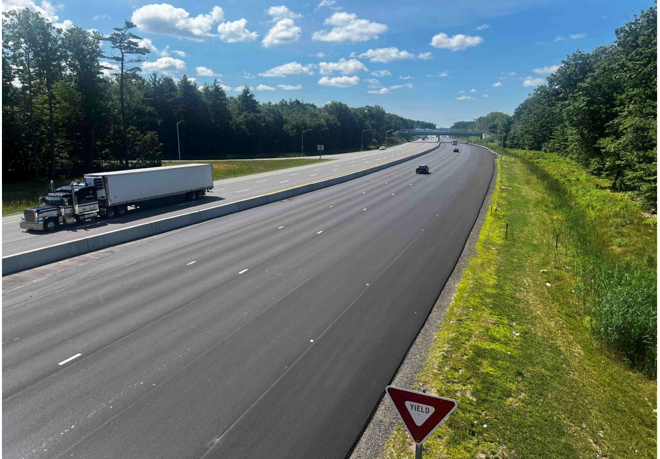
Looking south from Exit 47, all lanes have been surfaced paved.
