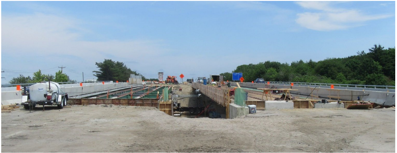
MCCR bridges phase 2
