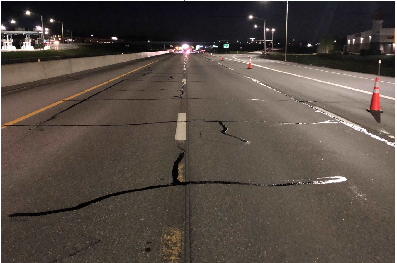
Looking north at Exit 45 after crews crack sealed the existing pavement
