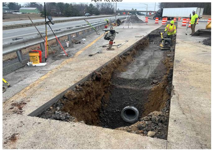
Looking south as the contractor backfills over a new drain line for the new fuel island.
