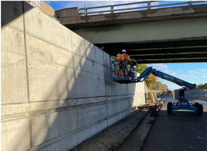
A crew touches up the concrete surfaces on the soil nail wall. Contractor: Sargent Corporation Bid Amount: \$41,922,810.00
