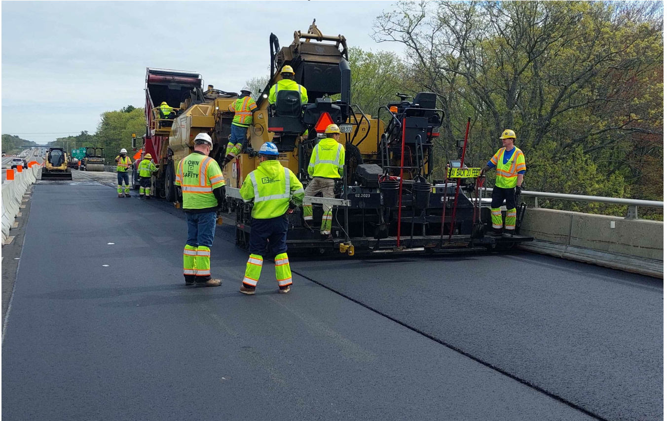
Pike Industries paving the B&M railroad bridge as part of this phase of the contract
