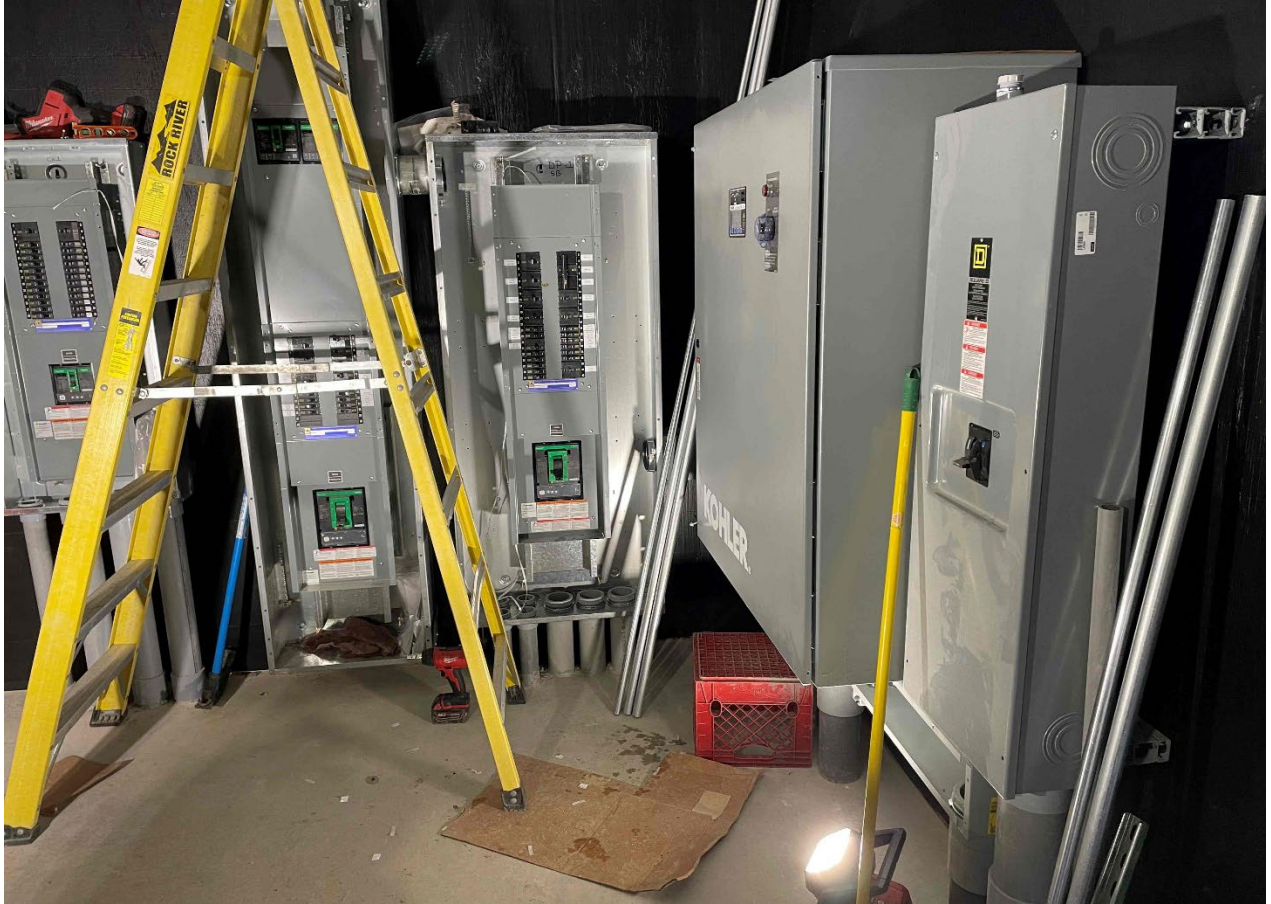
The southbound administration building power panels under construction.
