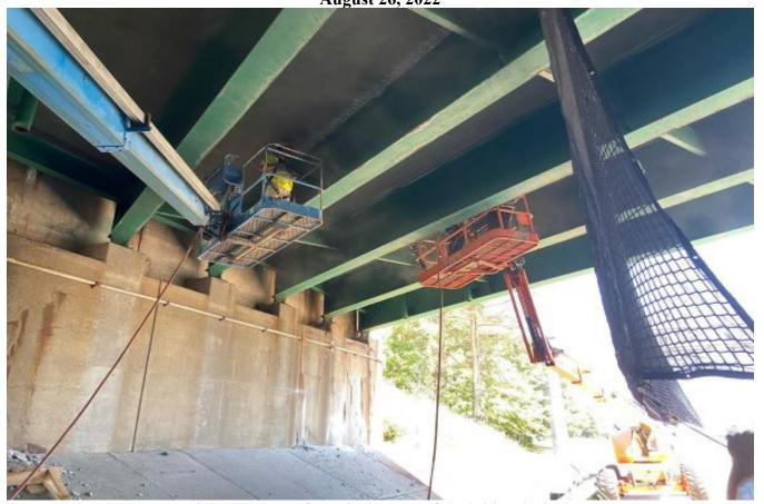
Crews work to remove loose concrete from the bottom of the bridge deck along Route 236.
